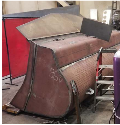
Stulz 8000 Cat 988 Rebuild 5/8 x 106 x 153 Floor
