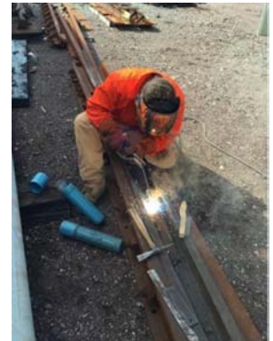
Applying Stulz XL to Frog Switch Point
