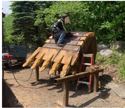
1" Wear Bars being welded to a 68" wide Stulz-Creusabro 8000 floor
