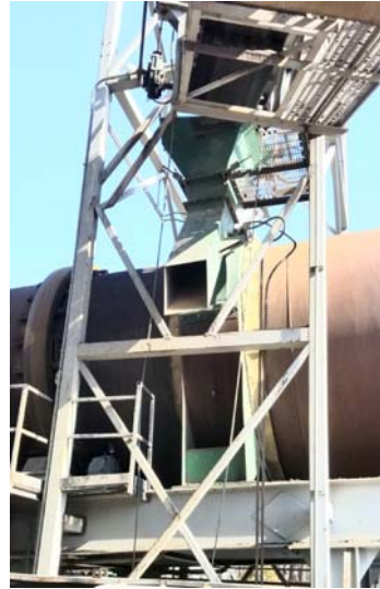
Stulz 8000 Rip-Rap Collar Installed 2016
