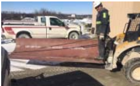
Ready to install a 3/8" 4800 Liner for a 980G
