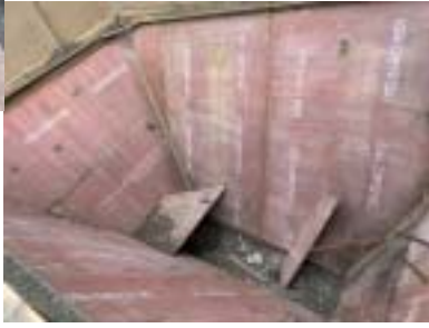
Lining 12 Bins with 4800 at a New Jersey Asphalt Plant
